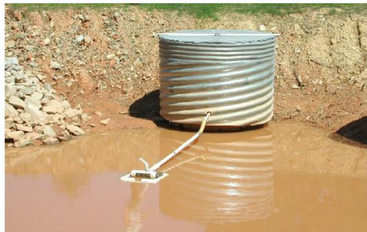
Figure 7.31-10B Floating Skimmer Installation
