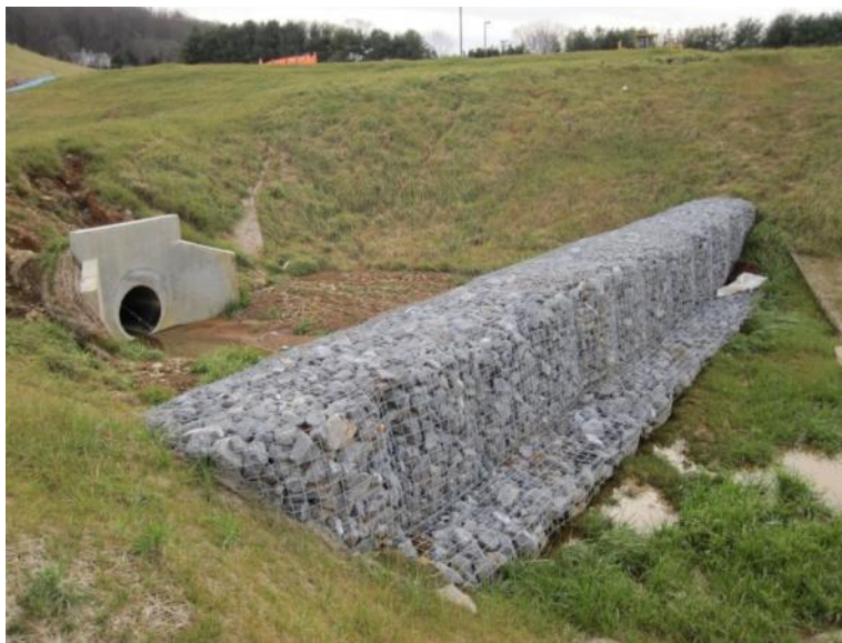
Figure 7.31-2C Forebay with Porous Berm (Gabion Rock)
